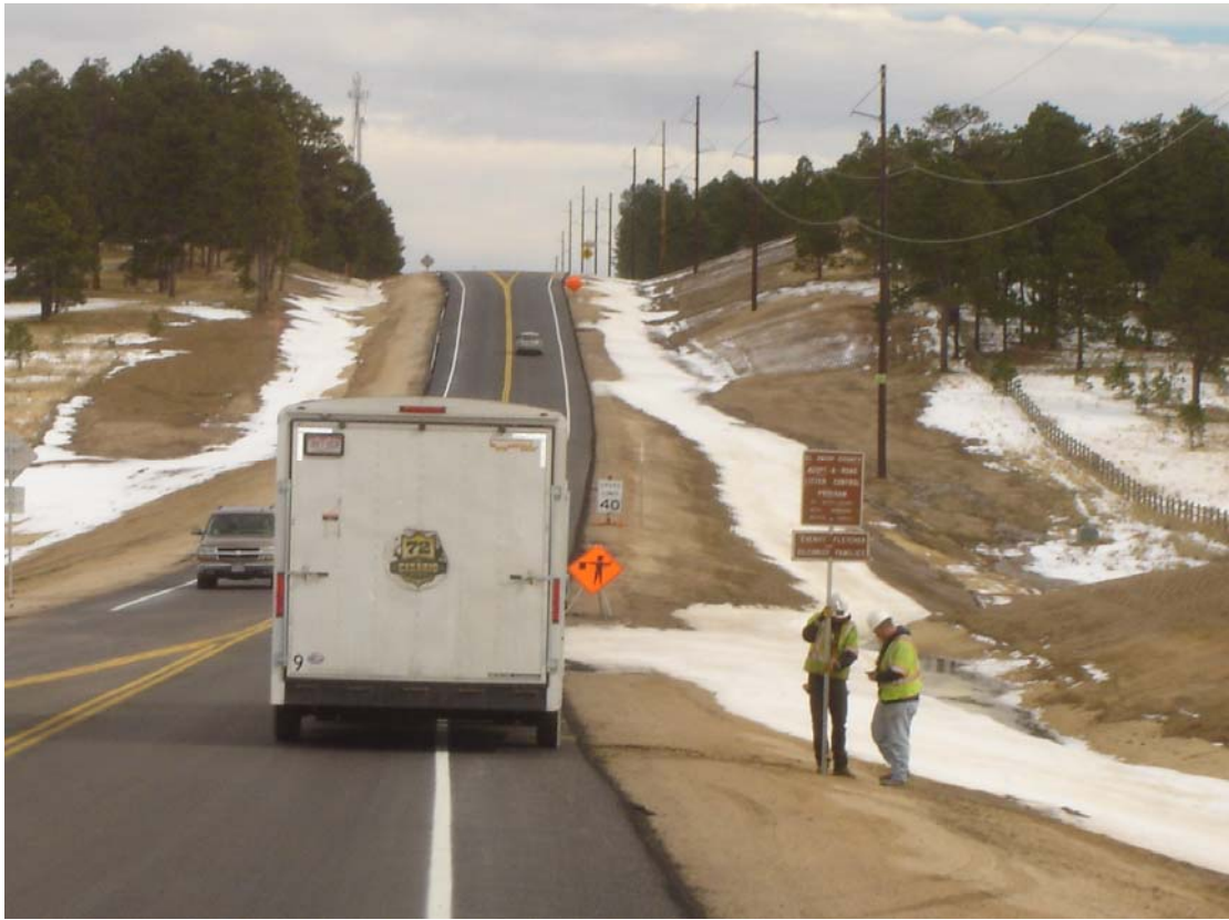
Workzone Permanent Sign Installation – November 2011
