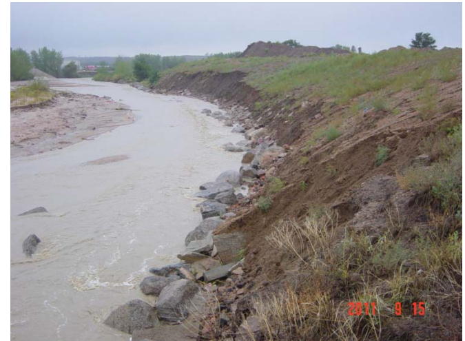
Erosion at Sand Creek ( private development)
