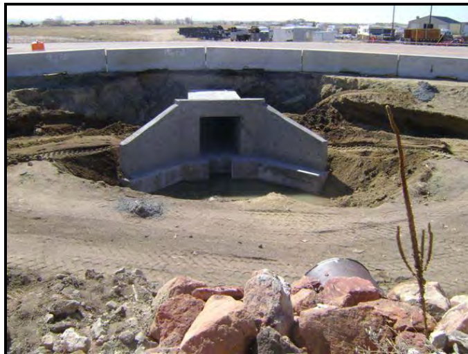
4'x4' reinforced Concrete Box Culvert extension at HWY 24
