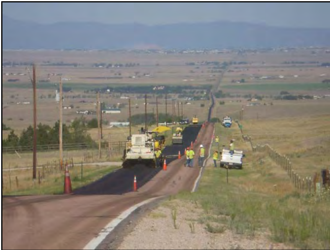
Asphalt Overlay on Judge Orr Road
