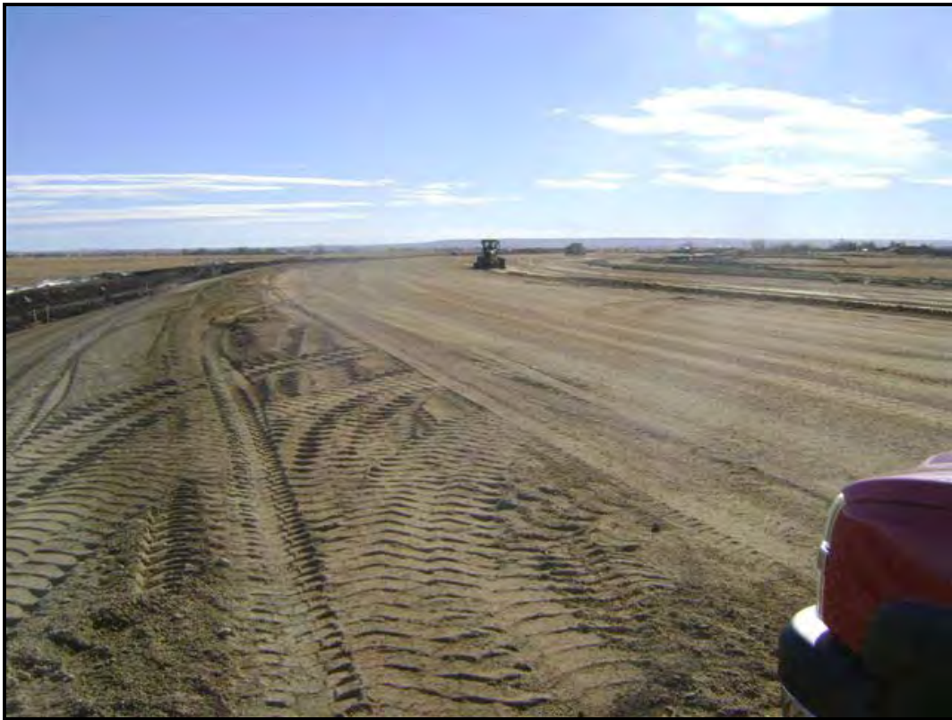
Grading Road Platform at Stapleton Road (West)
