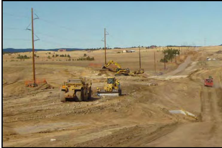
Roadway Construction looking west along Hodgen Road
